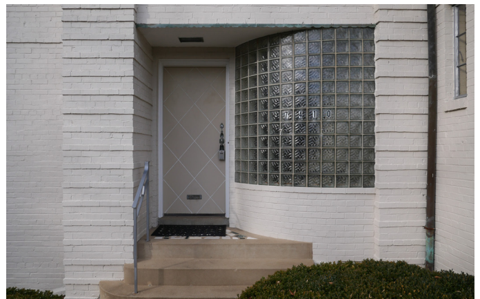
Figure 11: View of the front (east) elevation, 2020. The façade features a sweeping curved glass block wall that leads to the recessed main door. Source: Historic Preservation Program.
