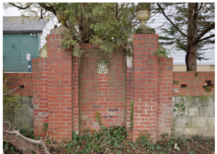
Figure 12: Detailed view of the brick and concrete block retaining wall. Source: Historic Preservation Program.
