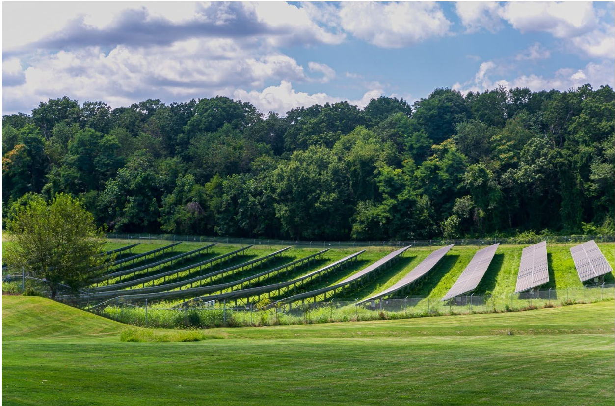
Solar array at South Germantown Recreation Park
