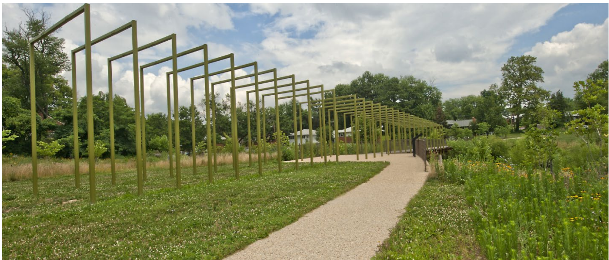
Evans Parkway Neighborhood Park renovation
