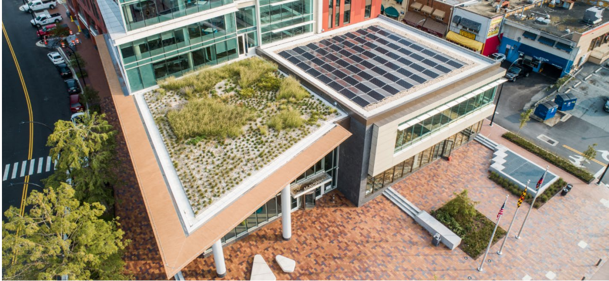
Lower-level green roof and solar array at Wheaton Headquarters
