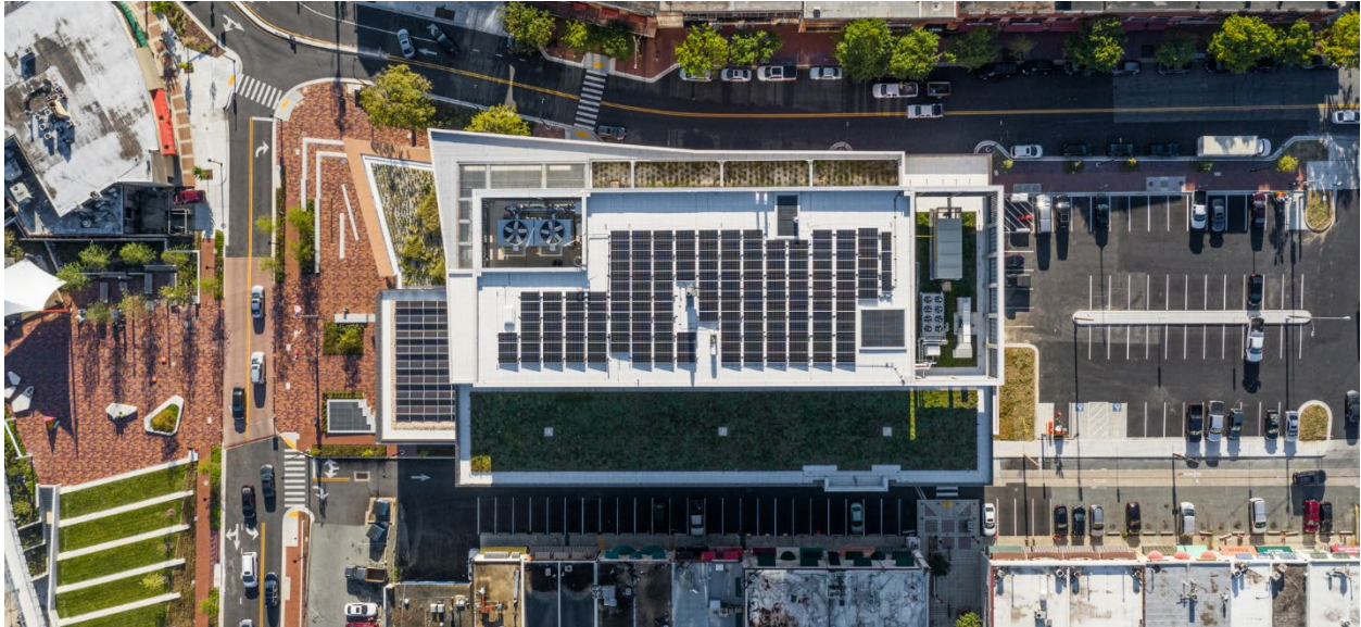
Solar and green roof at Wheaton Headquarters building
