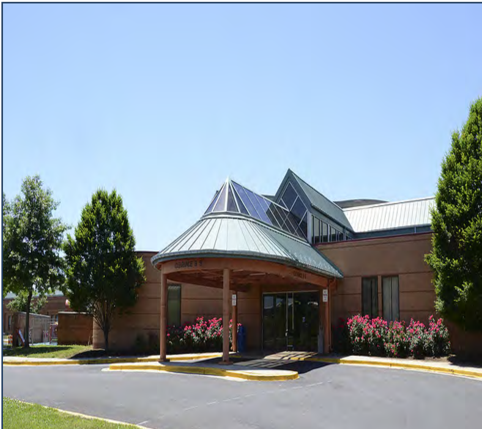
Exterior View of entrance to Largo Kettering Community Center
