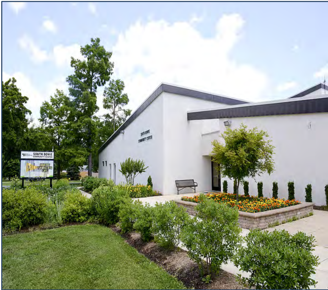
Exterior view of South Bowie Community Center
