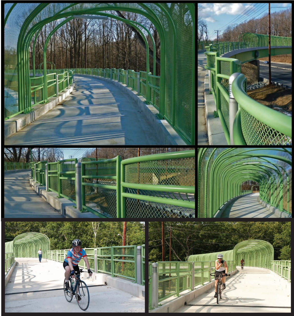
The Rock Creek Trail Pedestrian Bridge provides safe crossing of Viers Mill Road for trail users and community members.
