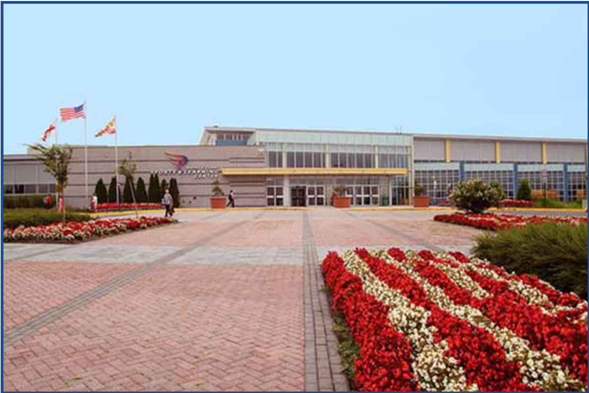
Exterior view of the Prince George's Sports & Learning Complex.
