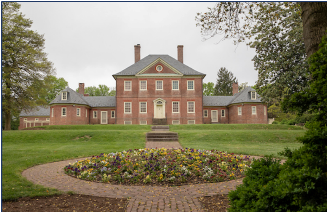
Exterior view of historic Montpelier Mansion
