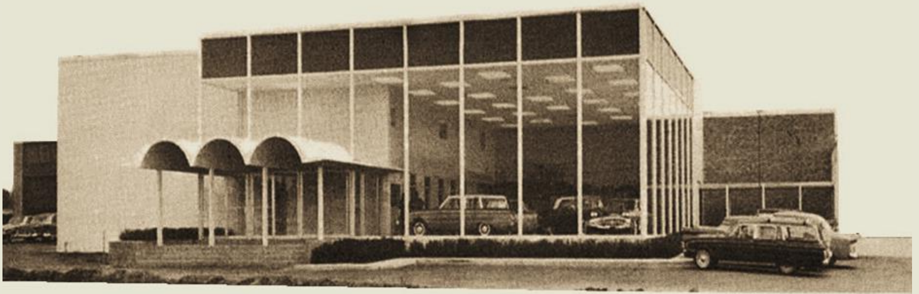
Above: Palmer Ford Showroom, Jamestown Road, John S. Samperton & Associates, 1960. (Demolished 1990) Courtesy Hyattsville: Our Hometown
